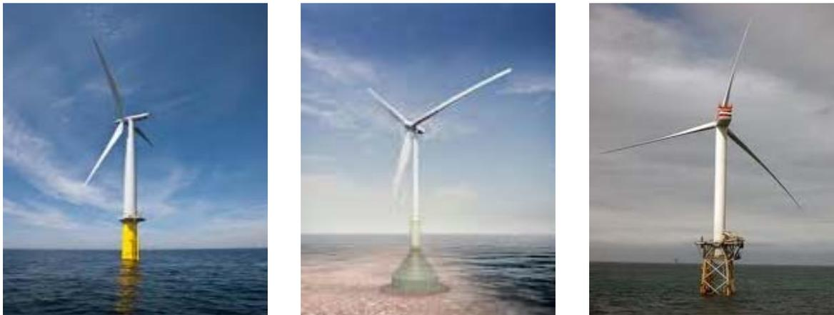
**Fig. 9** Prototype (a) monopile wind turbine and (b) gravity base wind turbine and (c) jacket type wind turbine (Musial and Butterfield (2006))
