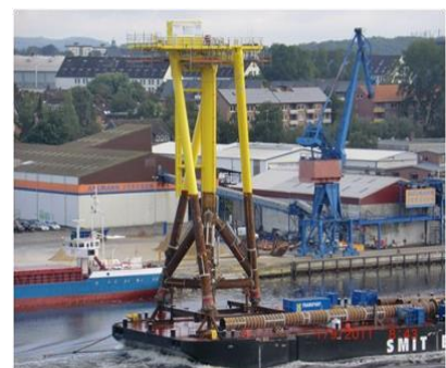
Fig. 14 Transportation and installation of a twisted jacket
