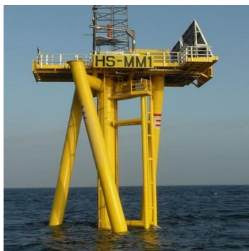
Fig. 5 Twisted jacket deployed in Hornsea (UK)
