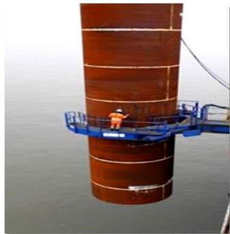
Fig. 1 Mono pile foundation
