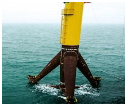
Fig. 3 Tripod foundation
