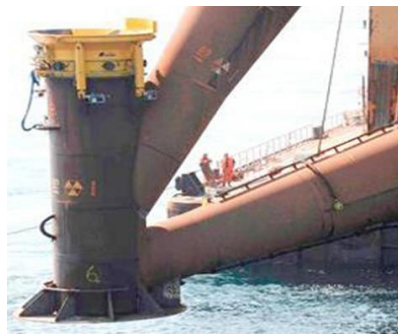
Fig. 13 Pile sleeve on a tripod foundation
