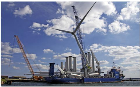
Fig. 10 Crane barge used for wind turbine installation
