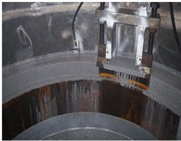
Fig. 15 Grouting material in mono pile foundation. Densit [25]
