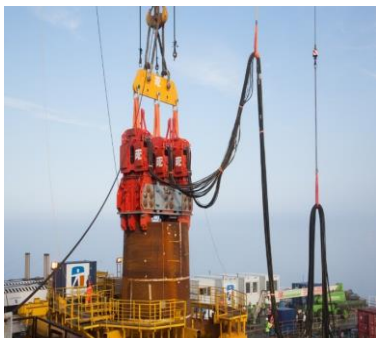
Fig. 12 Hydraulic hammer driving Mono pile to seabed
