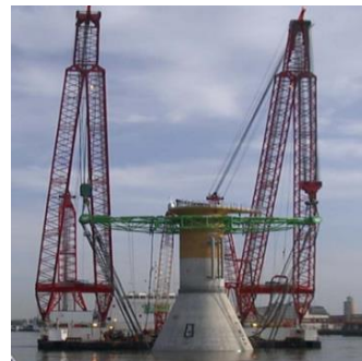
Fig. 2 Gravity-based foundation
