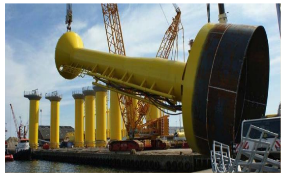
Fig. 6 Suction bucket structure (Photo: Dong Energy)
