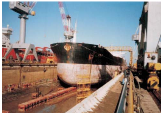
Figure 10 MT Ist, Docking No VII; Wetted surface condition before high pressure washing
